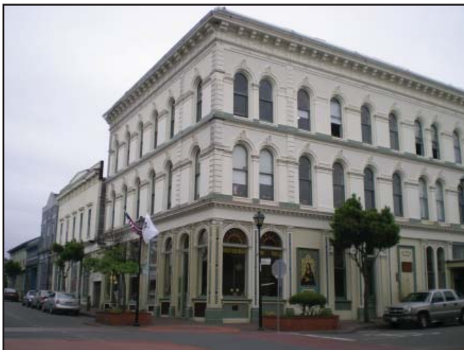
Commercial Buildings in Old Town Eureka
